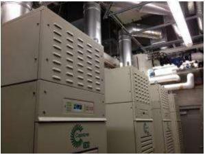
Microturbine CHP system installed in University of Toledo's Green Data Center. The system will be capable of providing 100 percent of the data center's critical electric and cooling needs.
